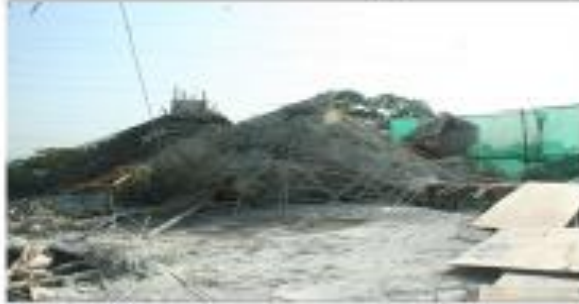
Collapsed form-work
