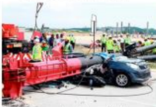
Car crushed by a fallen piling rig.
