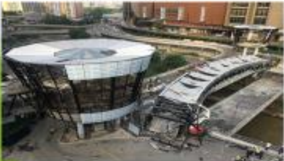
Collapsed steel bridge section
