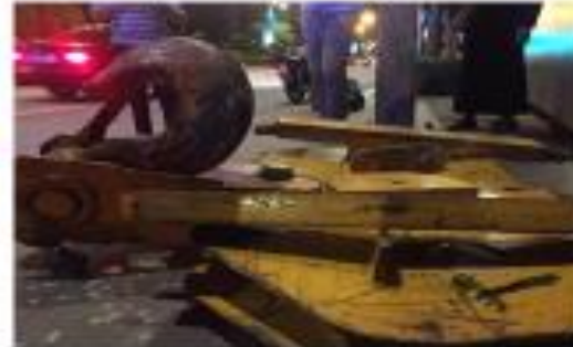
Lifting hook detached
