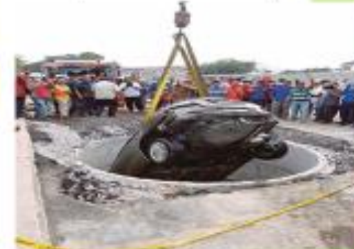
Car drove into an unprotected concrete shaft in the road
